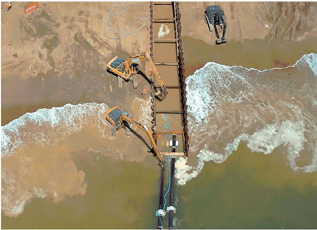
Figure 23 – Works at the landing point, RTE, Saint Nazaire, France.
