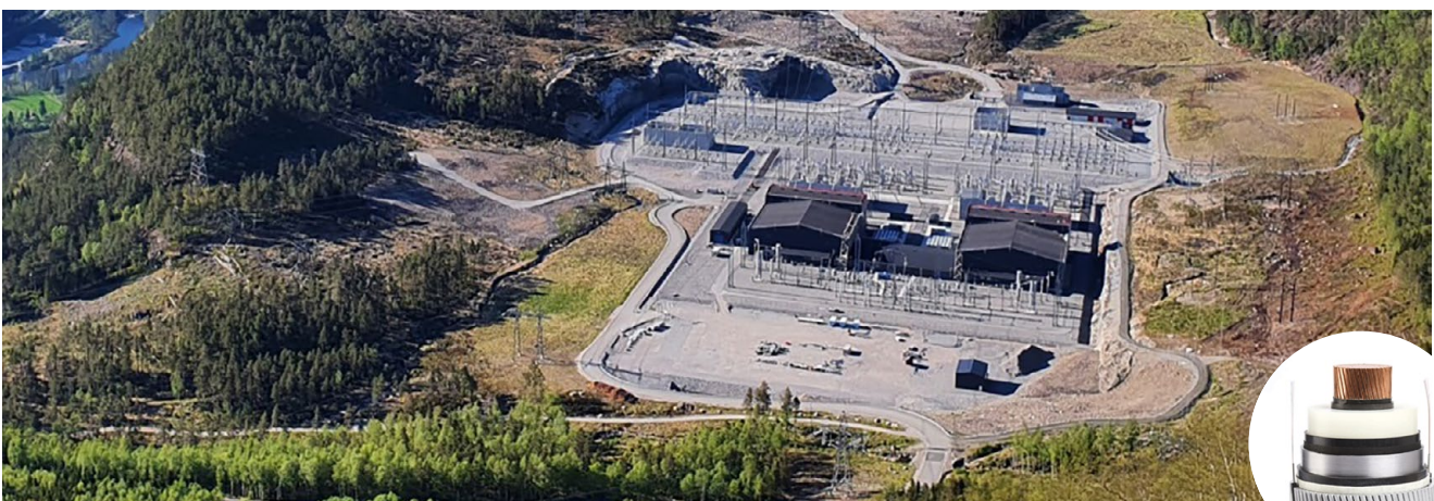
Figure 25 – 525 kV onshore converter station (Statnett, Tonstad, Norway) and onshore 525 kV cable (NKT).
