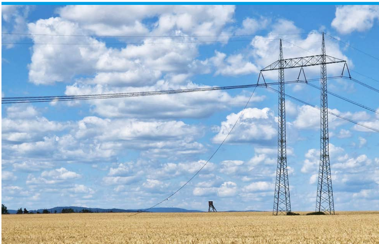
Figure 3.25: Photo of the fallen conductor
