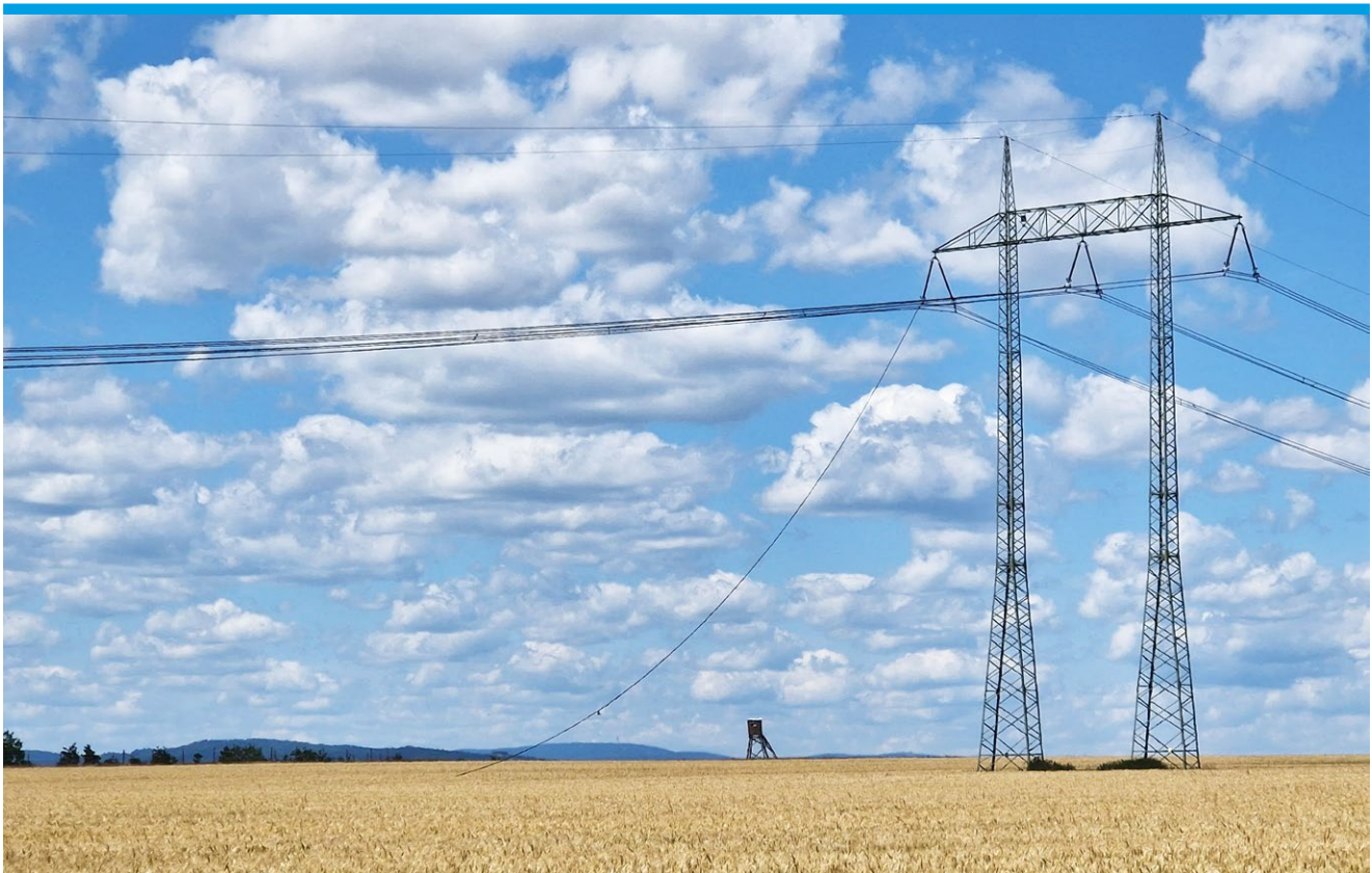
Figure 3.25: Photo of the fallen conductor
