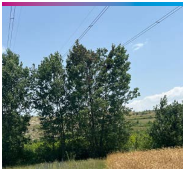
Figure 60: Picture of the area of the short circuit
